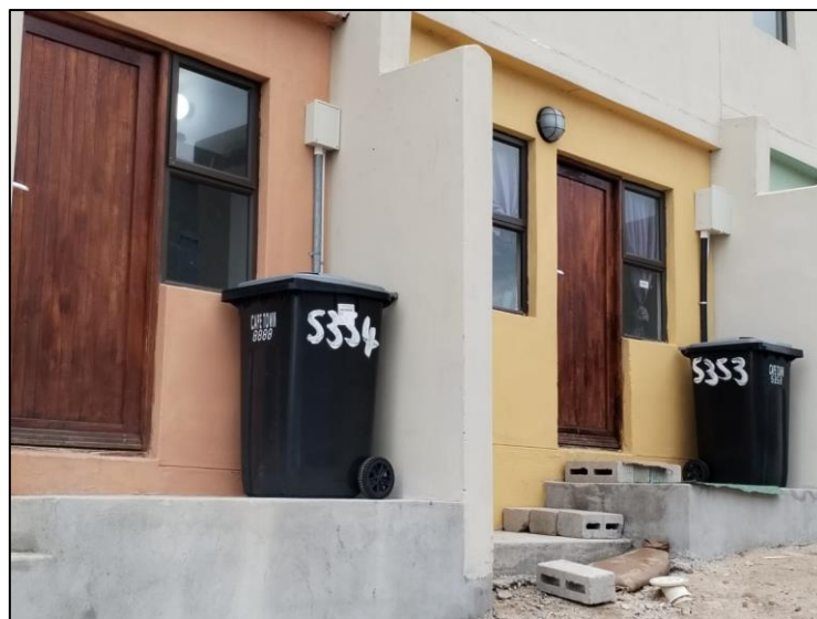
Figure 5. Lack of baboon-proofing measures at Dido Valley Housing Project.
